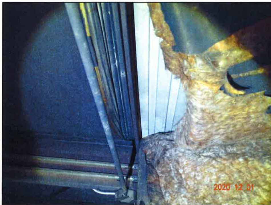
Photo 8: Underside of roof galvanized deck appeared generally in fair condition.
