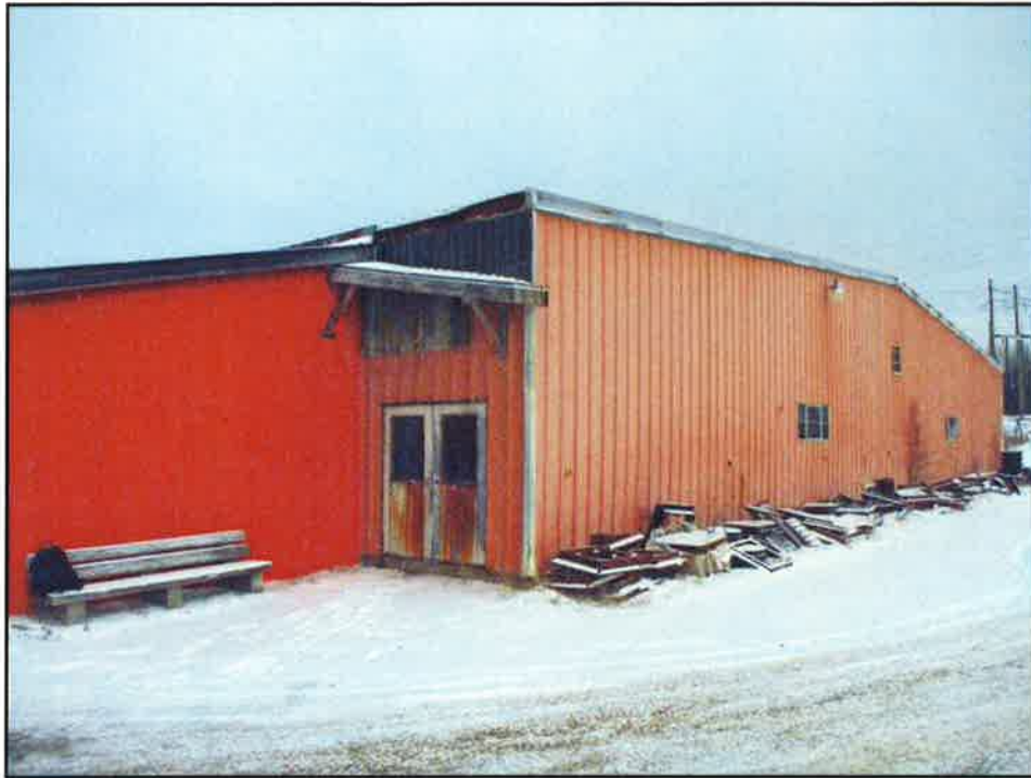
Photo 1: Public Works Garage located at 1 Dunfield Road, Kirkland Lake, Ontario.
