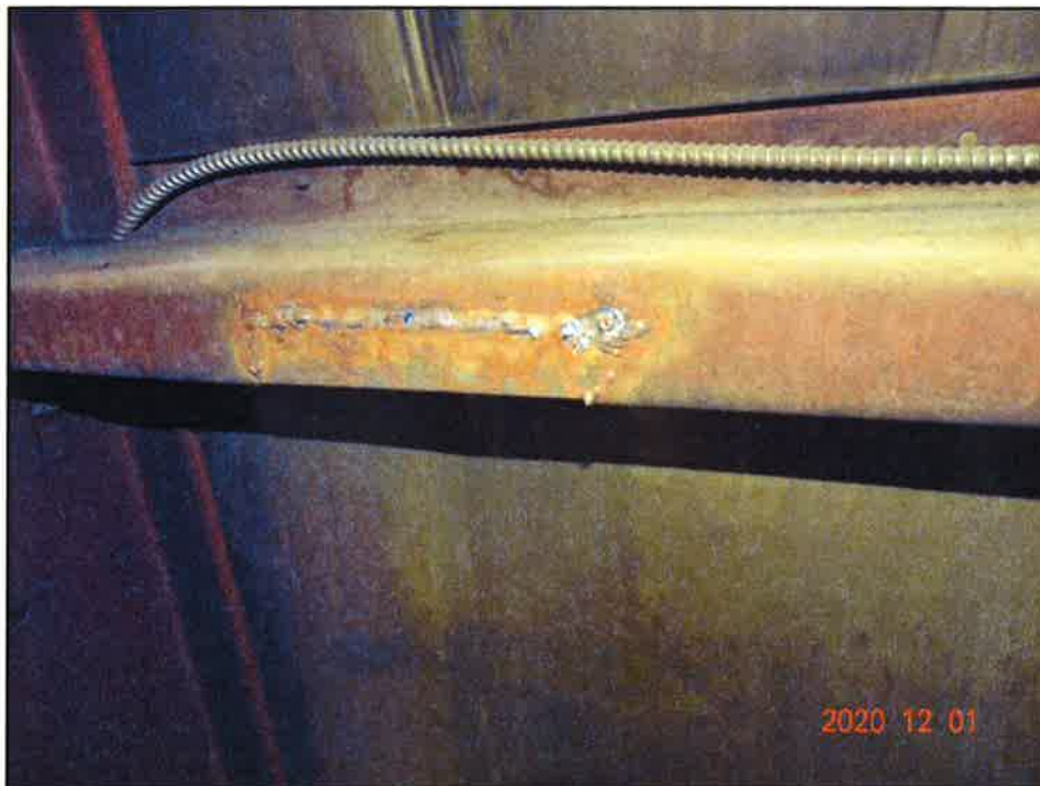
Photo 10: Coupon repair at wall girt with incomplete joint penetration weld and requires coating with zinc rich primer.
